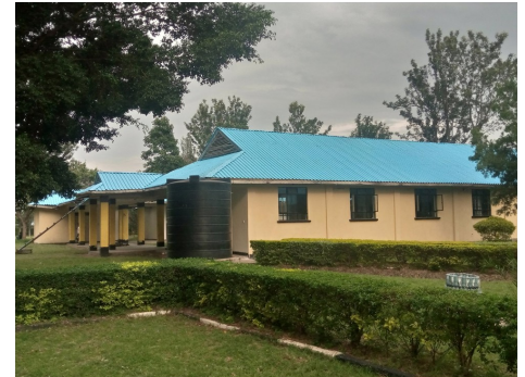
A section of KEWI Kisumu Campus during the ongoing painting exercise.
