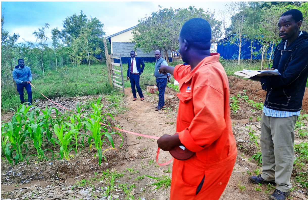
Kitui Campus team setting-out a SATO VIP latrines construction site.
