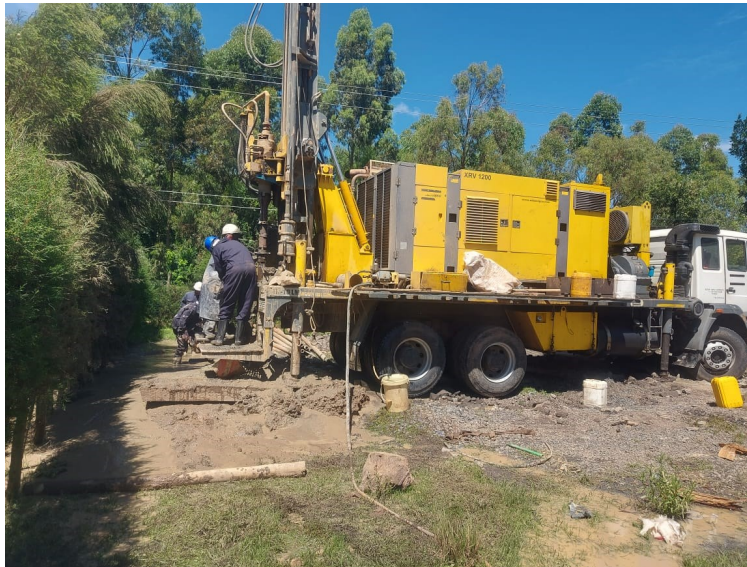
KEWI Drilling operations at a client's site.
