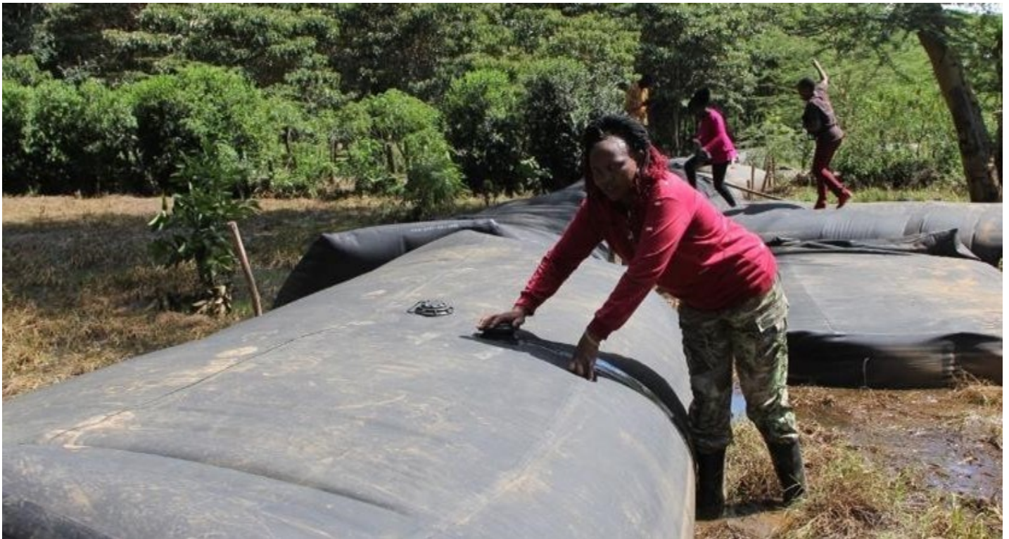
Illustration of a Slam dam, a flood control technology in use in Laikipia County. (Photo: Courtesy of Nation Media Group)
