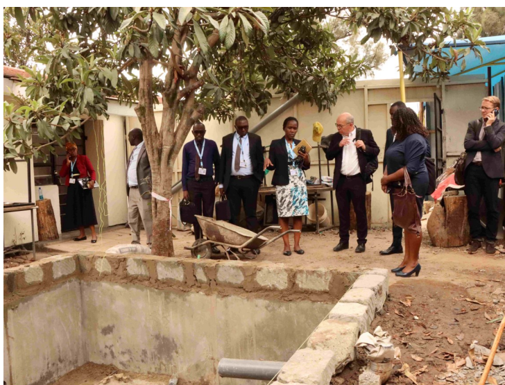
The team during the visit to the biogas plant construction site.
