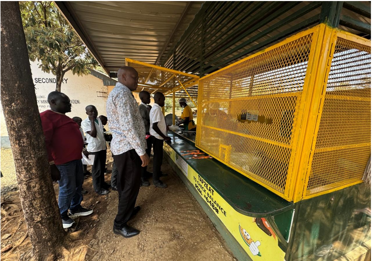
Dr. Letangule, EBS inspect a SATO toilet project at a school in the county. With him is Mr. Paul Rarieya, Head of Research Department at the institute.
