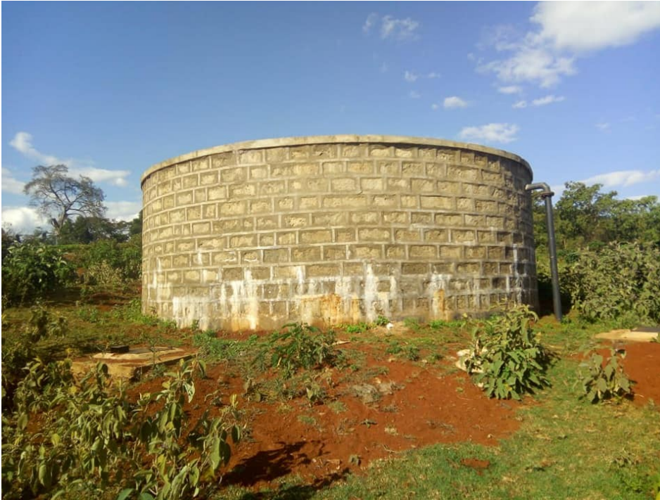
A masonry water tank and below villagers fetching water from a solar powered borehole.
