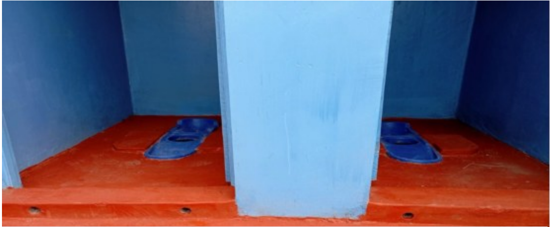
A SATO pans toilet. A study by KEWI researchers has shown that despite ongoing investments in water and sanitation infrastructure, many households still lack reliable water supplies and continue to use unimproved facilities that pose significant risks for disease transmission and environmental contamination.
