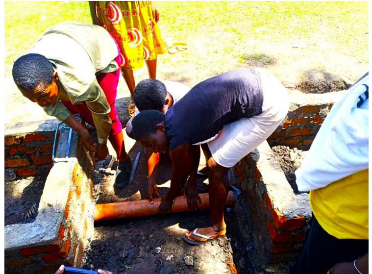
Plumbing and Pipefitting students during a practical lesson in Kisumu Campus
